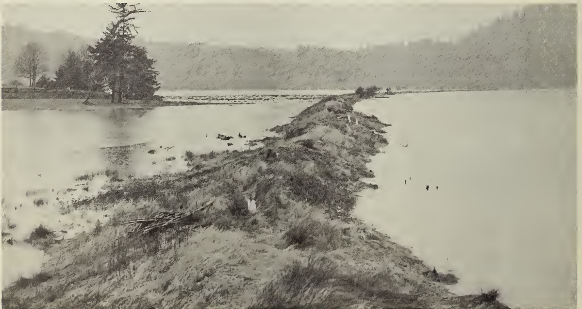
Photo 23.--Inadequate dikes and tidegates allow flooding along the Little Nestucca River in Oregon. SCS photo
